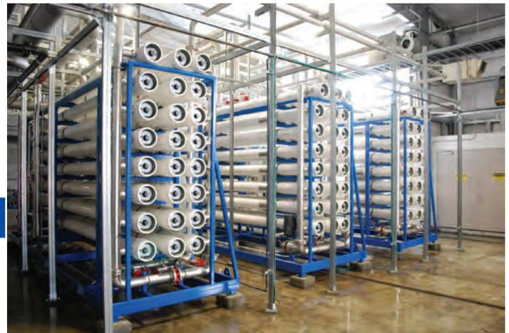
Full-scale UF (VersaFilter™) and RO systems built by WesTech Engineering, Inc. (photo credit WesTech. [www.westech-inc.com](http://www.westech-inc.com)).
